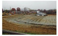
Site work is being completed, including filling in the valley behind the existing grandstands and the old hill in the northwest end zone. The existing stands will eventually be relocated.
